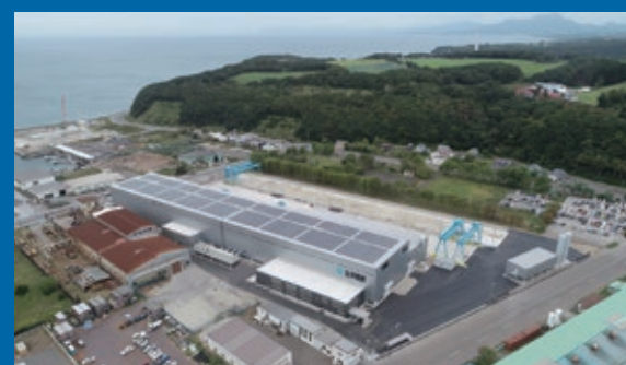
New Muroran Factory
