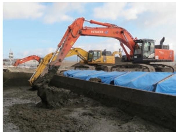
Mixing dredged soil and Calcia stabilized material with a backhoe
