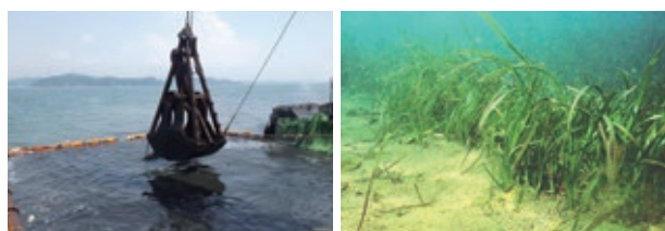
Shallow area and tidal flat development progress (injection of Calcia stabilized soil)
