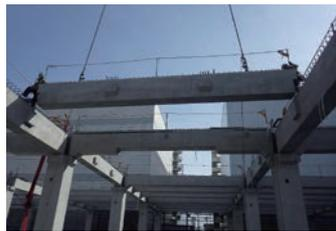
Installation of beams using PCa
