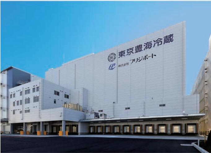
To address the labor shortage, we are implementing various labor-saving measures. In the construction of the Shin-Funabashi Logistics Center of Tokyo Toyomi Reizo Co., Ltd., the majority of the frame construction was precast method (PCa) to make on-site work safer and more efficient.
