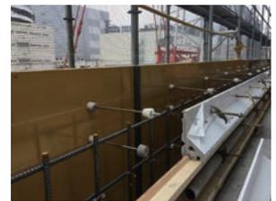
Parapets using the PCa method
