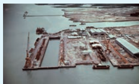
Undertook the construction of the pier at the Jurong Shipyard docks Foray into Singapore (1964)
