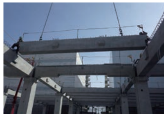
Installation of beams using PCa
