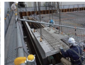
Berms using the PCa method
