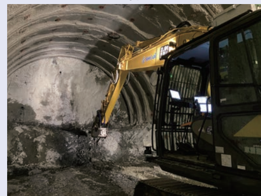
Unmanned and automatic drilling operation
