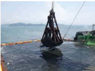
Shallow ground and intertidal flat development (injection of Calcia-stabilized soil)
