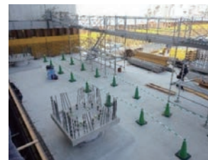
Upper part of seismic isolation foundation using the PCa method
