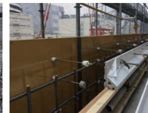
Parapets using the PCa method
