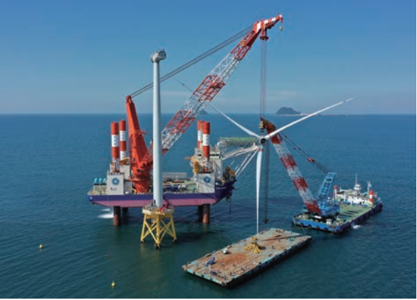
Kitakyushu Hibikinada offshore wind turbine removal (CP-8001 on the left)
