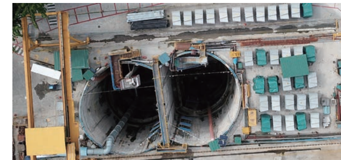
Consolidated shafts (Consolidation of shafts secures work space)
