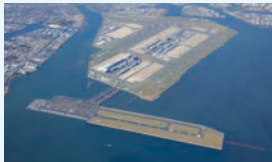
Opening of D-Runway of Tokyo International Airport (2010)
