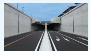
Completion of the Tokyo Port Umi no Mori Tunnel (2020)
