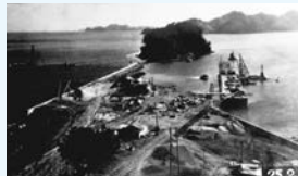
Contract awarded for construction of first large-scale quay walls and industrial facilities in the postwar era in Tsukumi Port, Oita Prefecture (1948)
