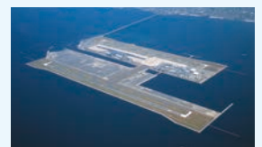
Contract awarded for phase I and phase II of construction of artificial island for Kansai International Airport (1986, 1999)
