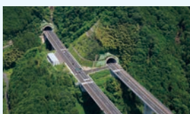
Completion of Kogouchi Tunnel of New Tomei Expressway (2005)
