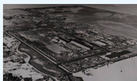
Contract awarded for construction of coastal industrial zone for NKK Corporation (currently JFE Engineering) in Fukuyama City (1961)
