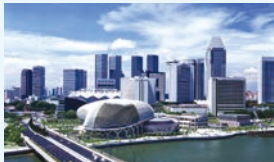
Completion of Esplanade-Theatres on the Bay in Singapore (2002)
