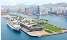
Completion of the Kai Tak Cruise Terminal (2013)
