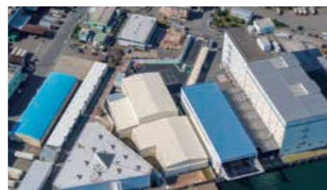
Yokohama Soil Recycling Center
