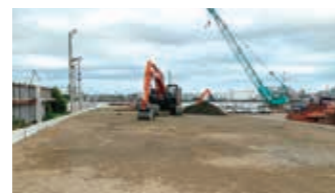
Temporary placement of tideland topsoil
