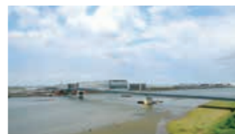
Situation after installation of bridge and restoration of tidal flat topsoil
