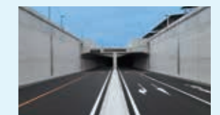
Completion of the Tokyo Port Umi no Mori Tunnel (2020)
