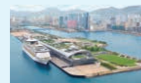
Completion of the Kai Tak Cruise Terminal (2013)
