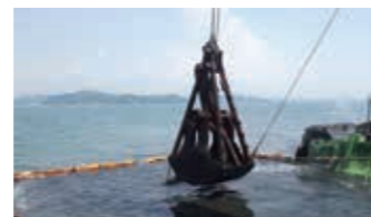
Shallow ground and intertidal flat development (injection of Calcia-stabilized soil)
