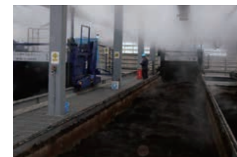
Inside the facility
