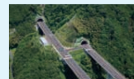
Completion of Kogouchi Tunnel of New Tomei Expressway (2005)
