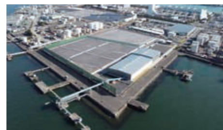
Nagoya Soil Recycling Center
