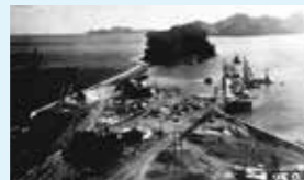
Contract awarded for construction of first large-scale quay walls and industrial facilities in the postwar era in Tsukumi Port, Oita Prefecture (1948)
