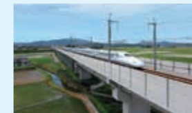
Completion of the Kyushu Shinkansen Tamanatsuru Bridge (2008)
