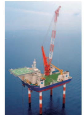
Completion of a multipurpose self-elevating platform, "CP-8001" (2018)
