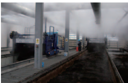
Inside the facility
