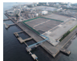
Nagoya Soil Recycling Center
