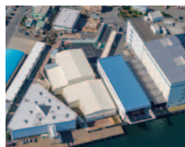
Yokohama Soil Recycling Center
