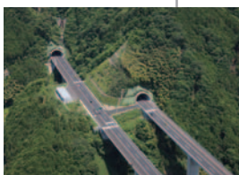
Completion of Kogouchi Tunnel of New Tomei Expressway (2005)
