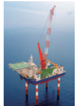
Completion of a multipurpose self-elevating platform, "CP-8001" (2018)
