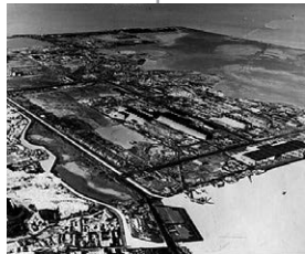
Contract awarded for construction of coastal industrial zone for Nippon Kokan Kabushiki Kaisha (currently JFE Engineering) in Fukuyama Prefecture (1961)
