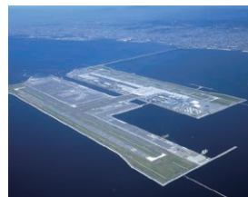
Contract awarded for phase I of construction of an artificial island for Kansai International Airport (1986)
