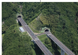
Completion of Kogouchi Tunnel of New Tomei Expressway (2005)
