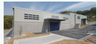
"Miki Biotech Co., Ltd." → a subsidiary company built a composting plant and began operating
