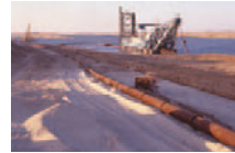
Extremely difficult Suez Canal repair work in progress
