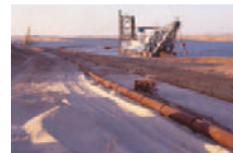
Extremely difficult Suez Canal repair work in progress
