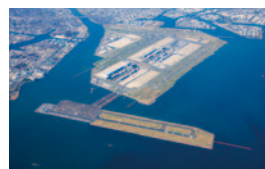
Major Japanese project - Tokyo International Airport Runway D
