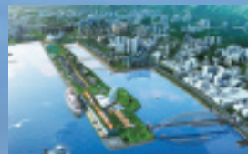
Construction work at the Kai Tak Cruise Terminal in Hong Kong
