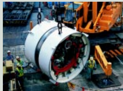
Asukayama main sewerage line project site
