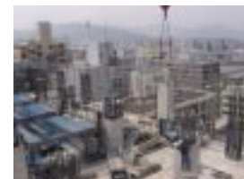
Pillar rods built in position
