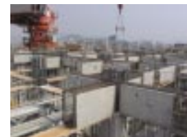
Completion of the framing work
