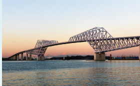
Completion of Tokyo Gate Bridge (2007)
