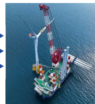
Wind turbine installation
