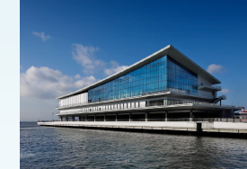
Completion of Tokyo International Cruise Terminal (2020)
