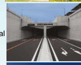
Completion of Tokyo Port Umi no Mori Tunnel (2020)
