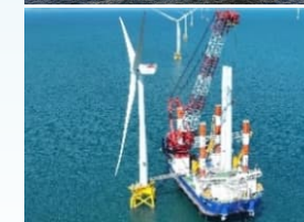
Completion of wind turbine foundations and marine works for the Kitakyushu Hibikinada Offshore Wind Power Project (2025)
