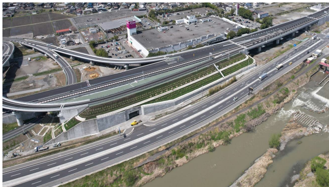
Tokai-Kanjo Expressway Takayanagi Construction Works (Mie, Completed in May 2025)
