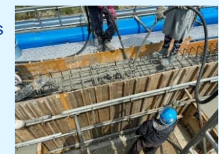
Placing of CELBIC-RA concrete
