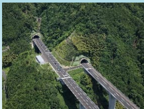
Completion of Kogouchi Tunnel of New Tomei Expressway (2005)
