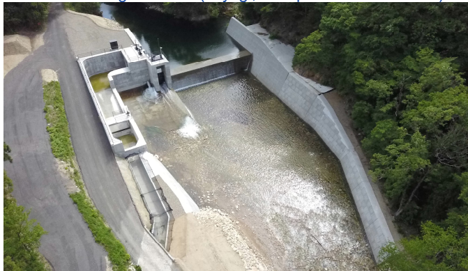
New Construction of Kurokoga River Hydroelectric Power Plant (Fukui, Completed in May 2025)
