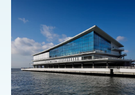
Completion of Tokyo International Cruise Terminal (2020)
