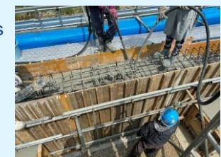
Placing of CELBIC-RA concrete
