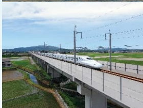
Completion of the Kyushu Shinkansen Tamanatsuru Bridge (2008)
