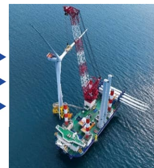
Wind turbine installation
