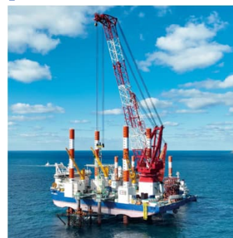
Foundation pile driving
