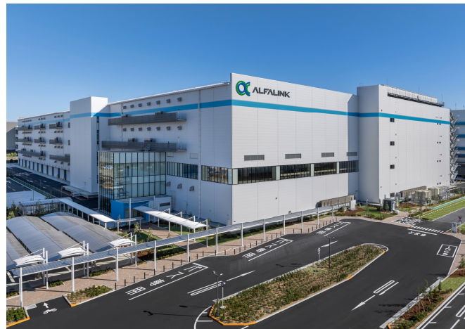
Amagasaki 4 Logistic Special Purpose Company, ALFALINK Amagasaki North Building (Hyogo, Completed in Oct. 2025)
