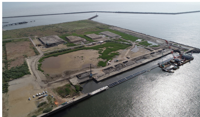
Construction Works of Quay (-12m) at Outer Port Area of Sakata Port (Yamagata, completed in May 2025)
