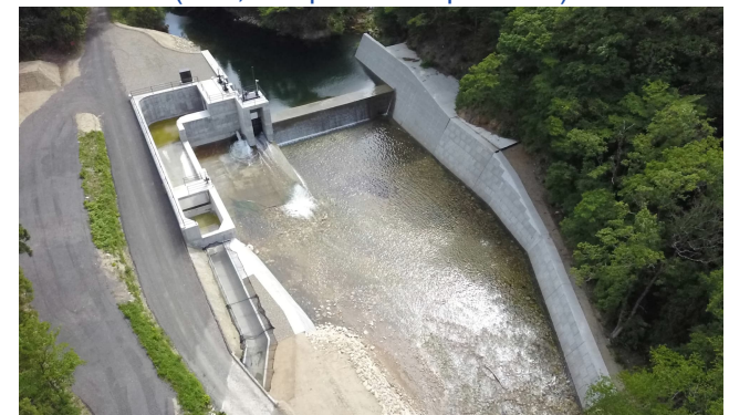
New Construction of Kuroko River Hydropower Plant (Fukui, completed in May 2025)
