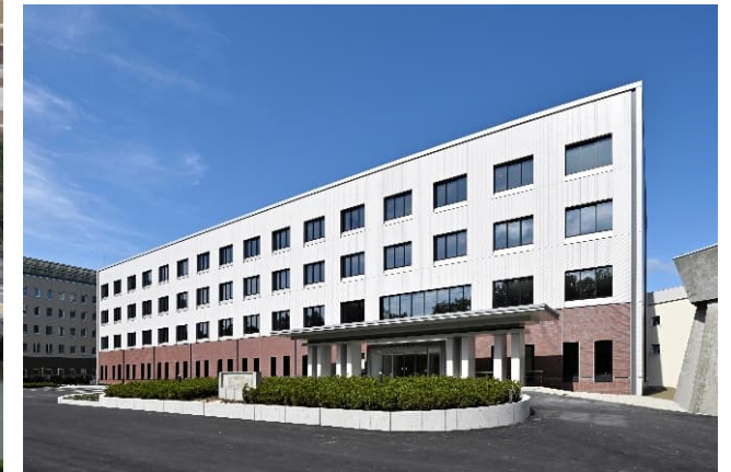
Hokkaido Police Academy, Main Building and Auditorium (Hokkaido, completed in September 2025)
