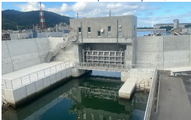
Wakayama Shimotsu Port Coast (Kainan area) Utsumi Sluice Gate and Seawall Construction (Wakayama Pref. completed in September 2024)
