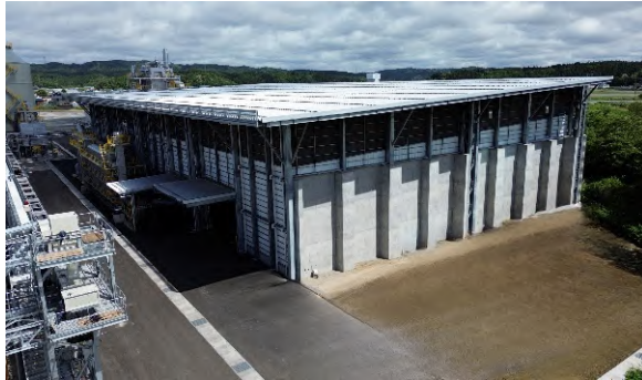
Chugoku Lumber Co., Ltd. Noshiro Factory, Construction of Fuel Storage etc. (Akita Pref. completed in July 2024)
