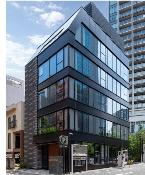
Hirakawacho LA BEFANA (Tokyo, completed in May 2024)
