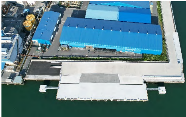
Construction of New Jetty for Onoken Shizuoka Center (Shizuoka Pref. completed in May 2024)
