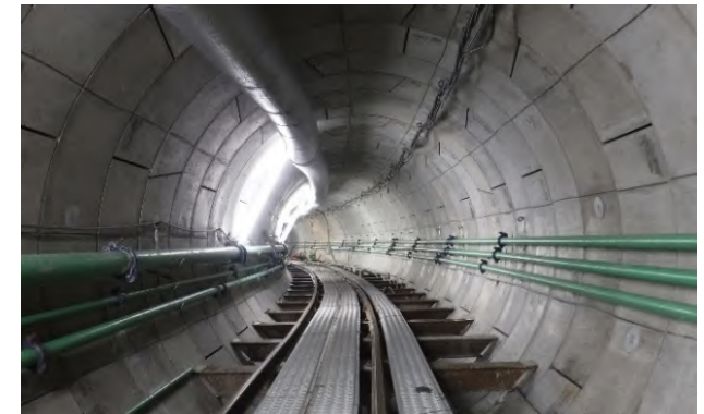
Branch Sewer Construction in Ota-ku, in the proximity of Naka-Ikegami 2-chome and Higashi Yukigaya 4-chome (Tokyo, completed March 2024)
