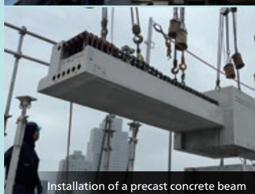
Installation of precast concrete underway at the first-floor slab level
