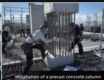
Installation of precast concrete underway at the first-floor slab level
