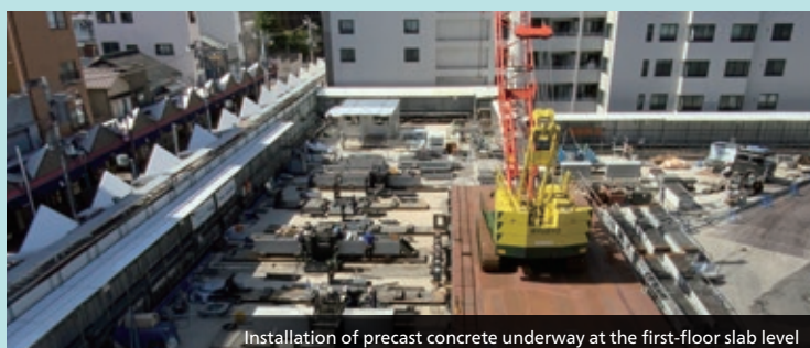
Installation of precast concrete underway at the first-floor slab level
