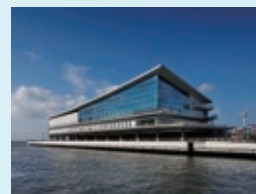
Completion of Tokyo International Cruise Terminal (2020)
