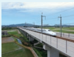
Completion of the Kyushu Shinkansen Tamanatsuru Bridge (2008)
