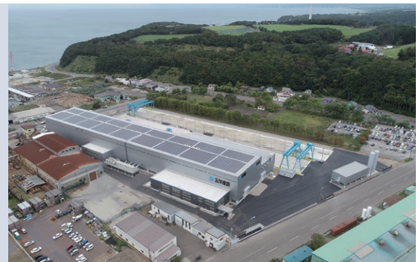
New Muroran Factory
