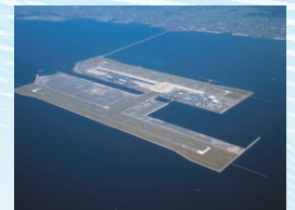
Contract awarded for phase I and phase II of construction of artificial island for Kansai International Airport (1986, 1999)
