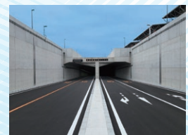
Completion of the Tokyo Port Umi no Mori Tunnel (2020)
