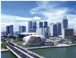
Completion of Esplanade-Theatres on the Bay in Singapore (2002)
