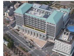
Completion of Kure City Hall (2015)
