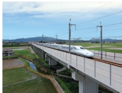
Completion of the Kyushu Shinkansen Tamanatsuru Bridge (2008)
