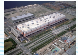
Completion of the World Cargo Distribution Center (1993)
