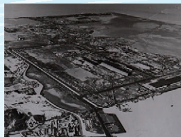
Contract awarded for construction of coastal industrial zone for NKK Corporation (currently JFE Engineering) in Fukuyama City (1961)
