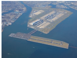
Opening of D-Runway of Tokyo International Airport (2010)
