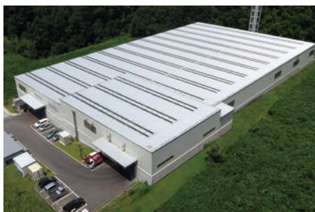
Panoramic view of the facility
