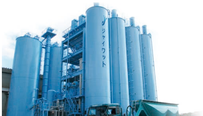
Panoramic view of the facility
