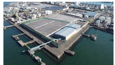
Nagoya Soil Recycling Center
