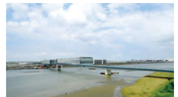
Situation after installation of bridge and restoration of tidal flat topsoil
