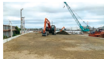
Temporary placement of tideland topsoil
