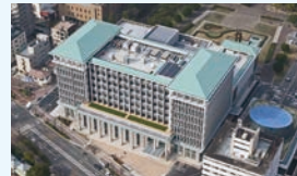
Completion of Kure City Hall(2015)
