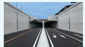
Completion of the Tokyo Port Umi no Mori Tunnel (2020)
