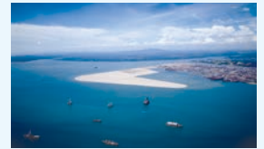
Contract awarded for Tuas Reclamation in Singapore (1984)
