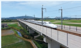
Completion of the Kyushu Shinkansen Tamanatsuru Bridge (2008)
