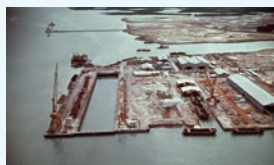
Undertook the construction of the pier at the Jurong Shipyard docks Foray into Singapore (1964)
