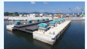
Completion of the Mirai Shipbuilding Yard (2019)
