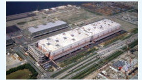
Completion of the World Cargo Distribution Center (1993)
