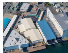
Yokohama Soil Recycling Center
