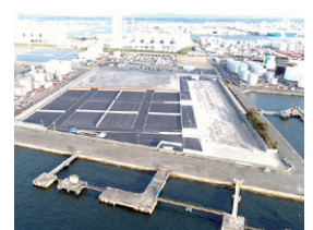
Nagoya Soil Recycling Center
