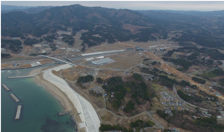
Progress of construction work (as of May 2018)
