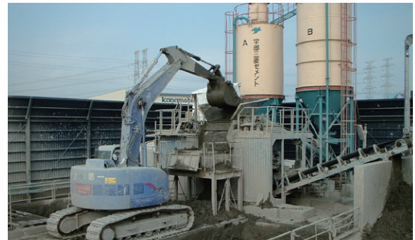
Sludge treatment plant
