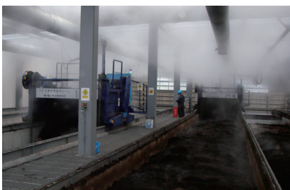
Inside the facility
