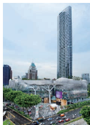
Construction work at the ION Orchard and the Orchard Residences in Singapore
