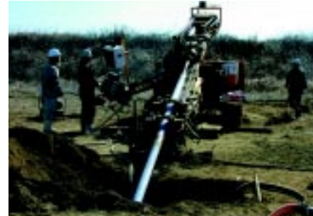
A drilling machine of bent drilling hole method
