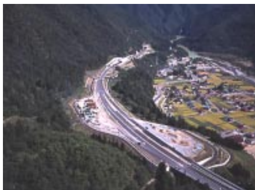
Shimoda Tunnel of Tokai-Hokuriku Expressway, Gifu
