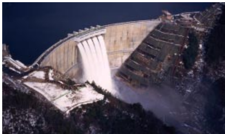
Nukui Dam, Hiroshima
