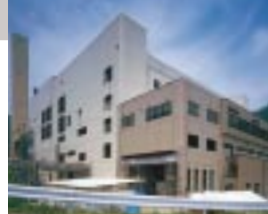
▶ Hitachi recycling and disposal center, Ibaraki
