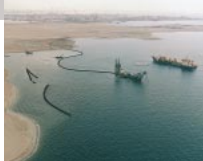
Reclamation of Jurong Island Phase 3B, Singapore
