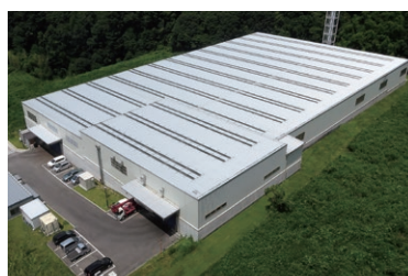
Panoramic view of the facility
