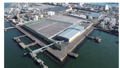
Nagoya Soil Recycling Center
