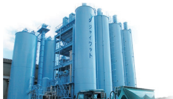
Panoramic view of the facility
