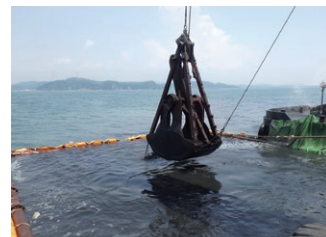
Shallow area and tidal flat development (injection of Calcia stabilized soil)
