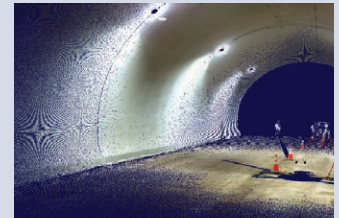
Point group data of lining surface collected by an autonomous four-legged walking robot
