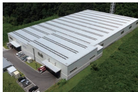
Panoramic view of the facility
