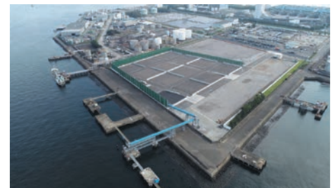
Nagoya Soil Recycling Center
