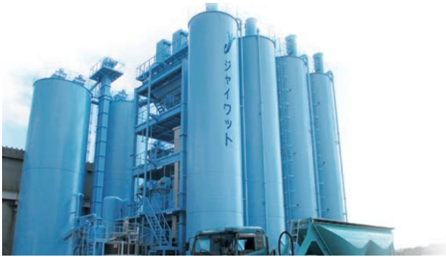
Panoramic view of the facility
