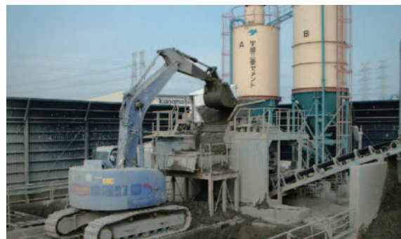
Sludge treatment plant
