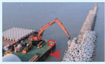
Realization of labor saving by managing the history of the installed blocks by using the underwater sonar fitted on the part shown in red in the photo
