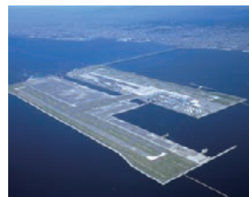
Contract awarded for phase I of construction of an artificial island for Kansai International Airport (1986)
