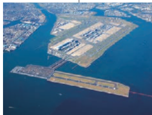
Opening of D-Runway of Tokyo International Airport (2010)
