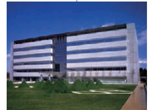
Completion of New Technology Institute in Nasushiobara City, Tochigi Prefecture (1994)
