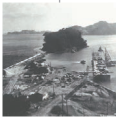
Contract awarded for construction of first large-scale quay walls and industrial facilities in the postwar era in Tsukumi Port, Oita Prefecture (1948)
