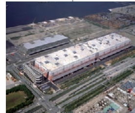
Completion of the World Cargo Distribution Center (1993)
