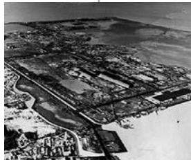
Contract awarded for construction of coastal industrial zone for Nippon Kokan Kabushiki Kaisha (currently JFE Engineering) in Fukuyama Prefecture (1961)
