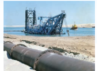
Cutter suction dredger "Suez"
