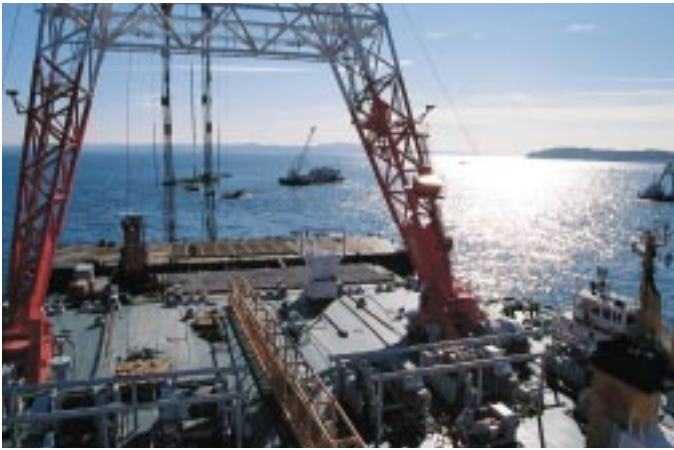
Hoisting work at Tokyo bay
