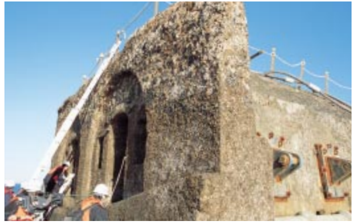
1,211-ton hoisted concrete structure
