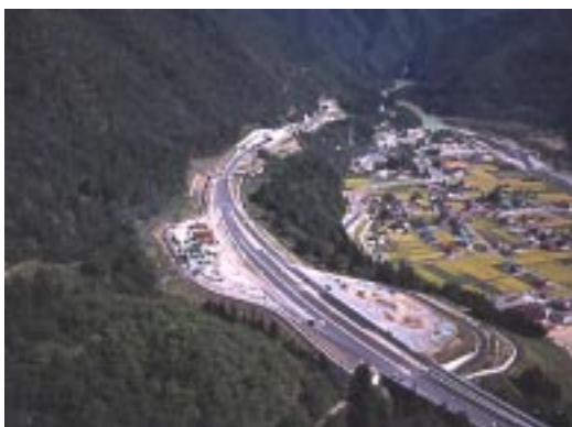
Shimoda Tunnel of Tokai-Hokuriku Expressway, Gifu
