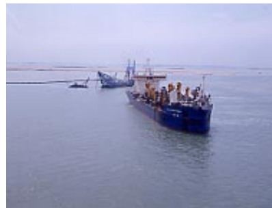
Queen of Penta-Ocean engaged in dredging work in Singapore
