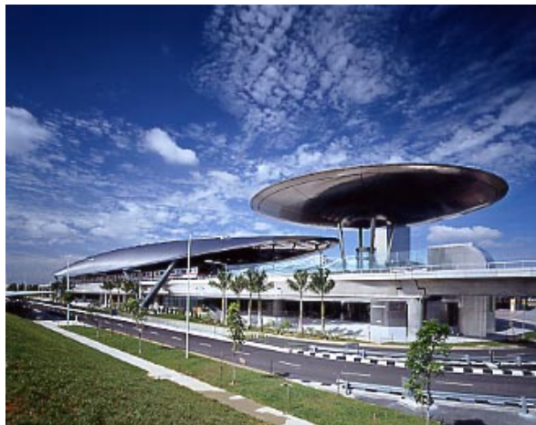
MRT502 Expo station on the Changi Airport line, Singapore (picture by courtesy of SMPT)
