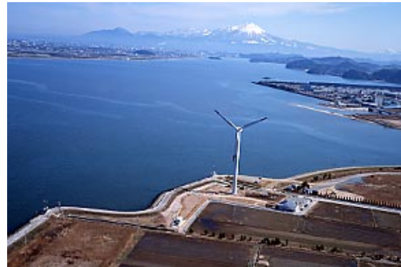
Yasugi wind power station, Shimane
