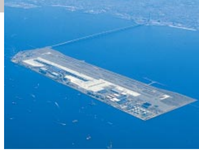
Kansai International Airport reclamation work Phase II, Osaka
