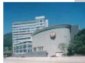
Hong Kong Academy of Medicine headquarters, Hong Kong
