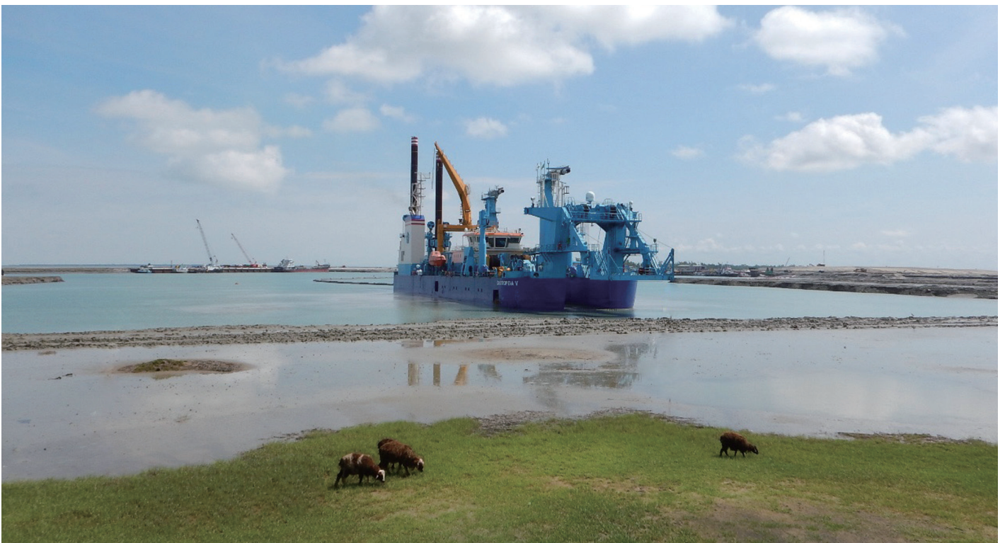
CASSIOPEIA V dredging in this project
